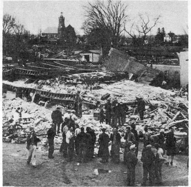
STORE DESTROYED BY TORNADO
