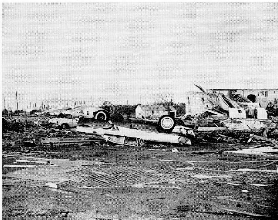
Destruction left by tornado that hit El Dorado, Kansas, on June 10, 1958.
